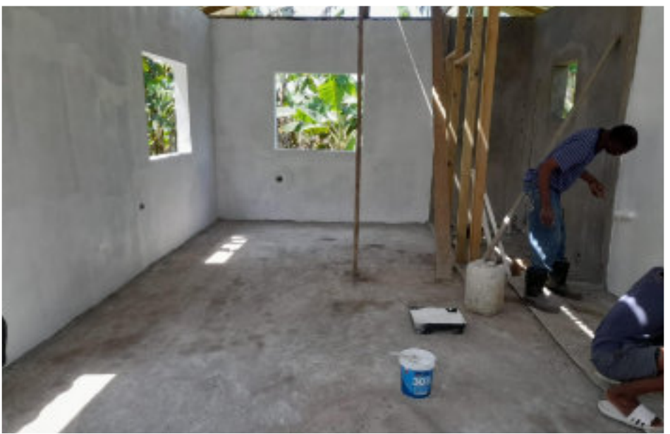
Members of the Lewis Store, St. Mary, built a house in April 2022, for Maud Kennedy an elderly member of the Clonmel community whose house was destroyed by fire.
