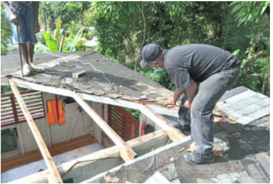
The Westmoreland Chapter of Men's and BEAMS continued their mission of serving others by taking on a house renovation project for a needy family on June 19 and July 1, 2022.
